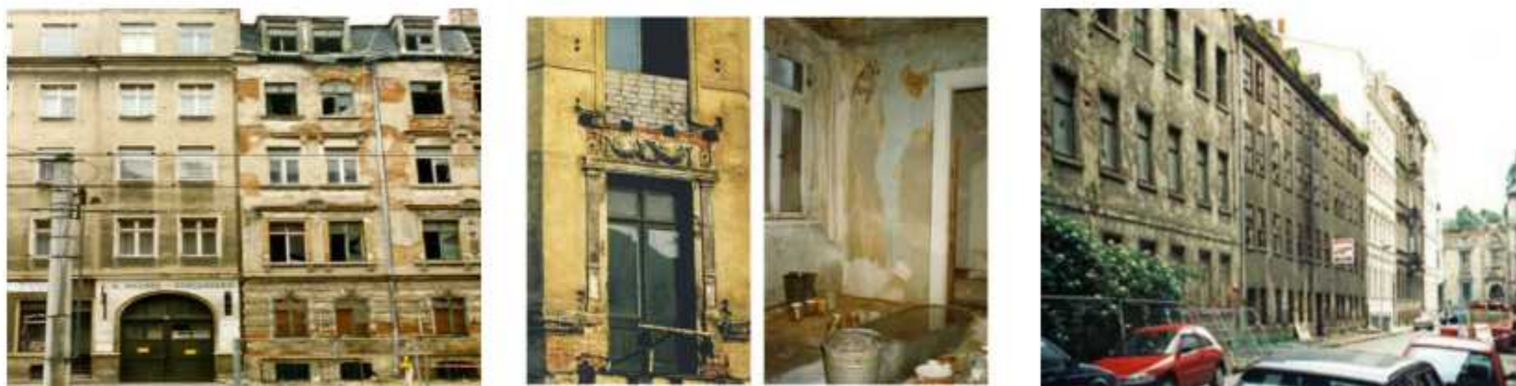
Figure 2 – Derelict houses at the end of the GDR period (1949-1989), Source: Stadt Leipzig (2017)
