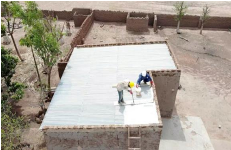
Application of cool roof coating
